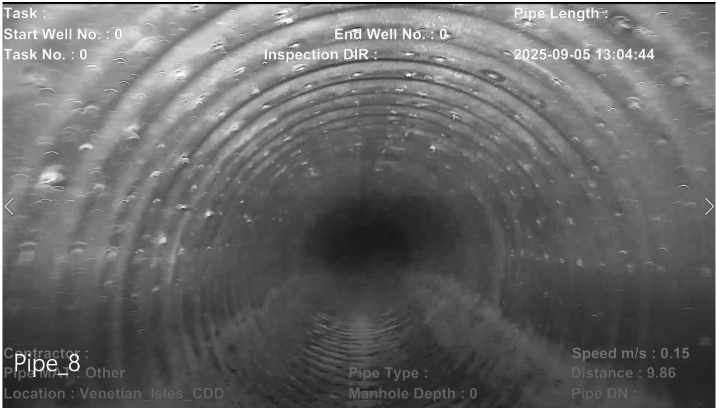
CCTV Crawler entered from S610 heading south, pipeline found in good condition.
