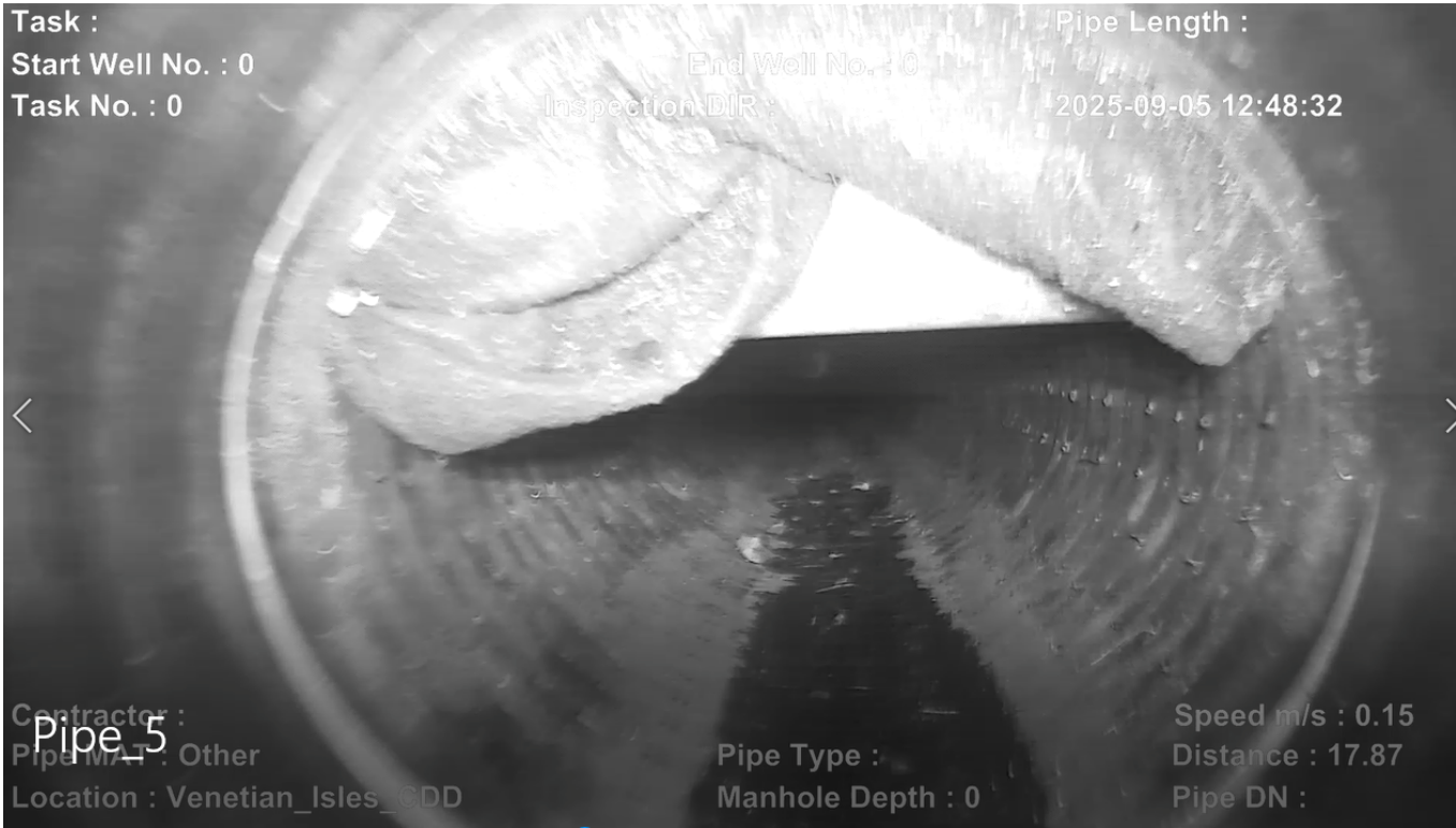
Sanitary sewer lateral crossing at approximately 58LF.
