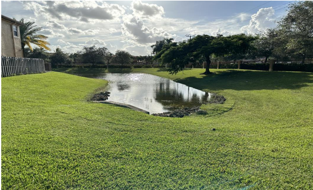
Figure 20: Bank erosion showing depression.
