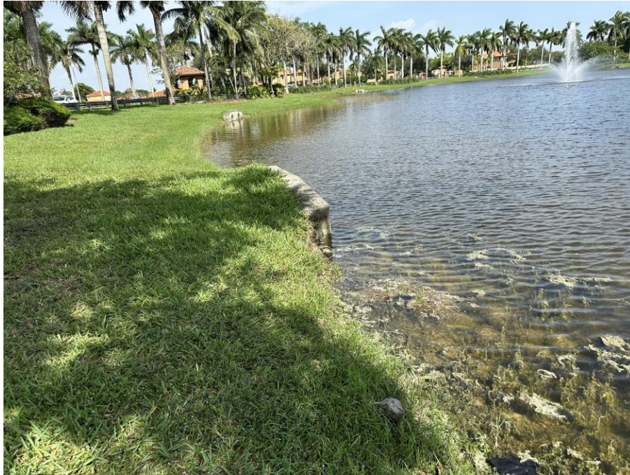
Figure 22: Slope is good; however, loss of land is shown.
