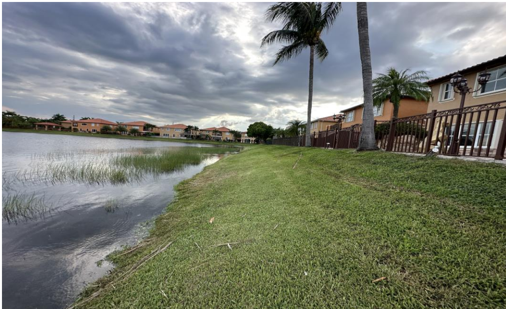
Figure 8: Bank erosion with uneven shoreline with a drop off at water's edge.
