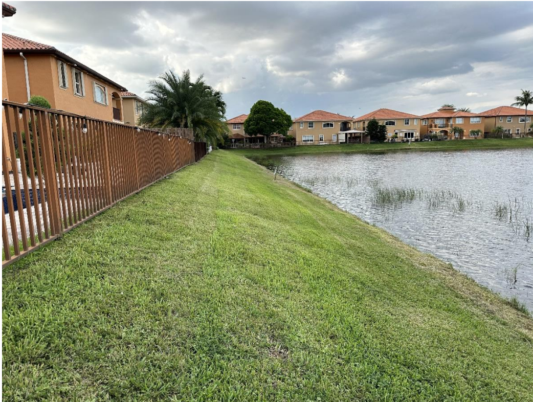
Figure 11: Steep slope with a drop off at the water's edge.
