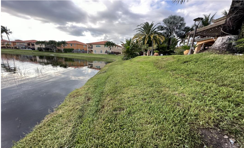
Figure 7: Bank erosion with steep drop from the top of the embankment.
