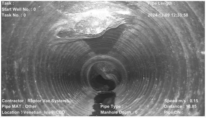
Significant blockage and collapse, S705 looking north.
