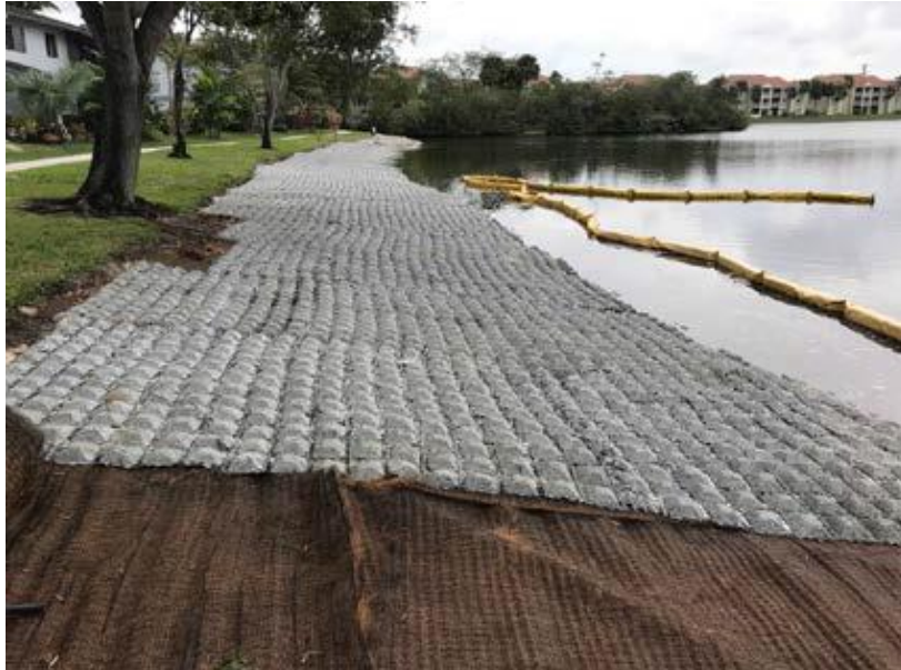
Figure 33: During Landshore's installation of Flexamat®
