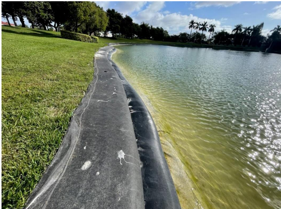
Figure 30: Example of EFT® Landshore's Installation
