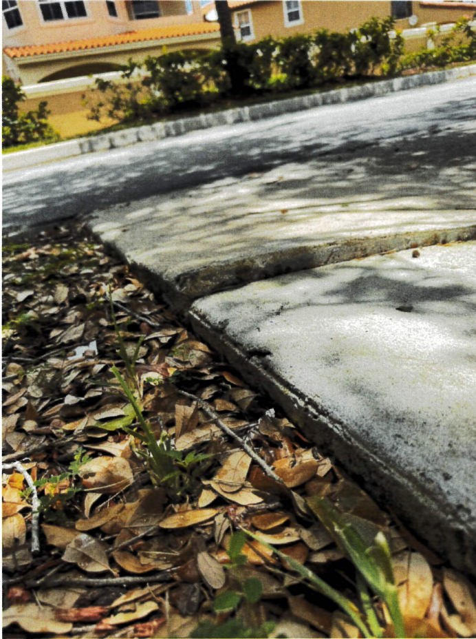
Storm Drain Concrete Repairs/Replacement
