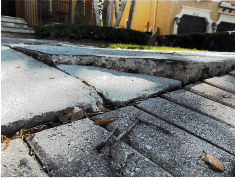
Sidewalk Slab Replacement
