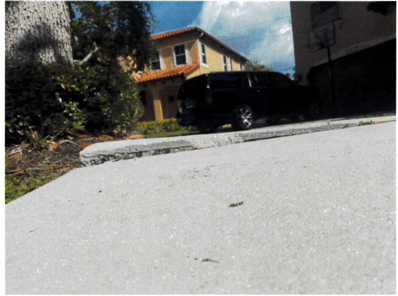
Sidewalk Slab Replacement
