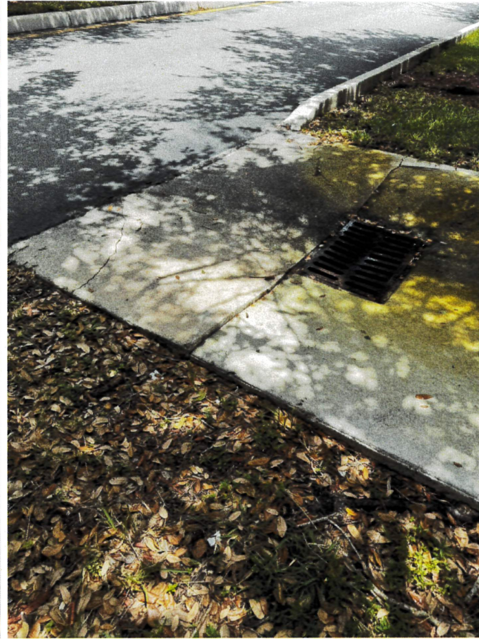
Storm Drain Concrete Repairs/Replacement
